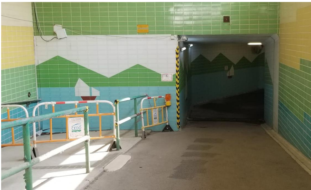
Photo 3 - Erection of site hoardings in unobtrusive colours
