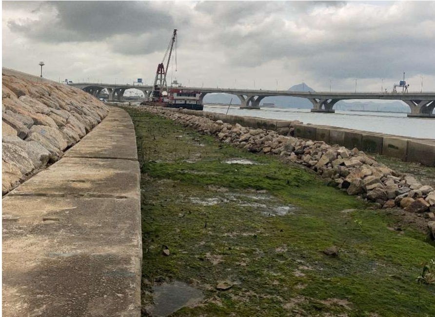
General View of Mangrove Eco-shoreline Upper Terrace
